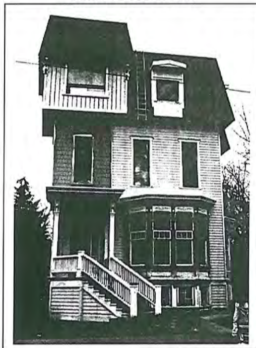
False mansard roof
