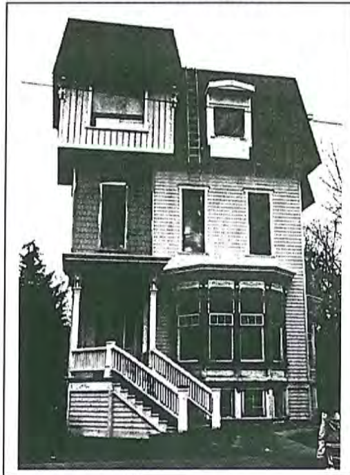
False mansard roof
